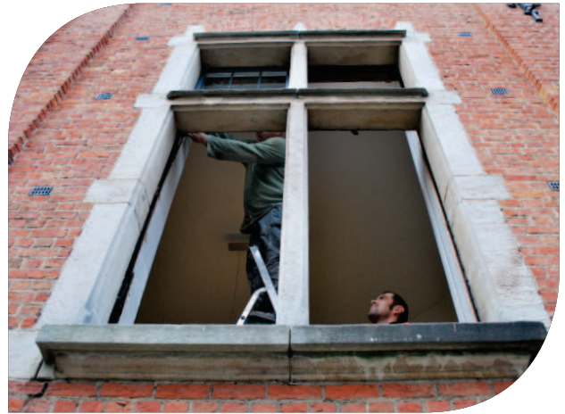
Replacing the windows of the CEER office
